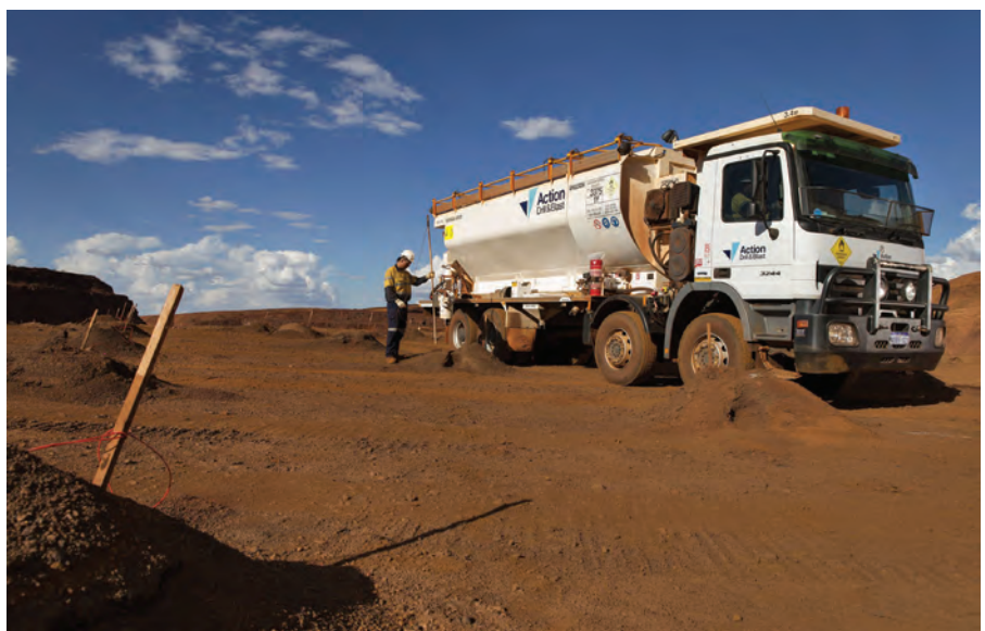
An Action Drill & Blast mobile processing unit in operation at a West Australian iron pre-project.
